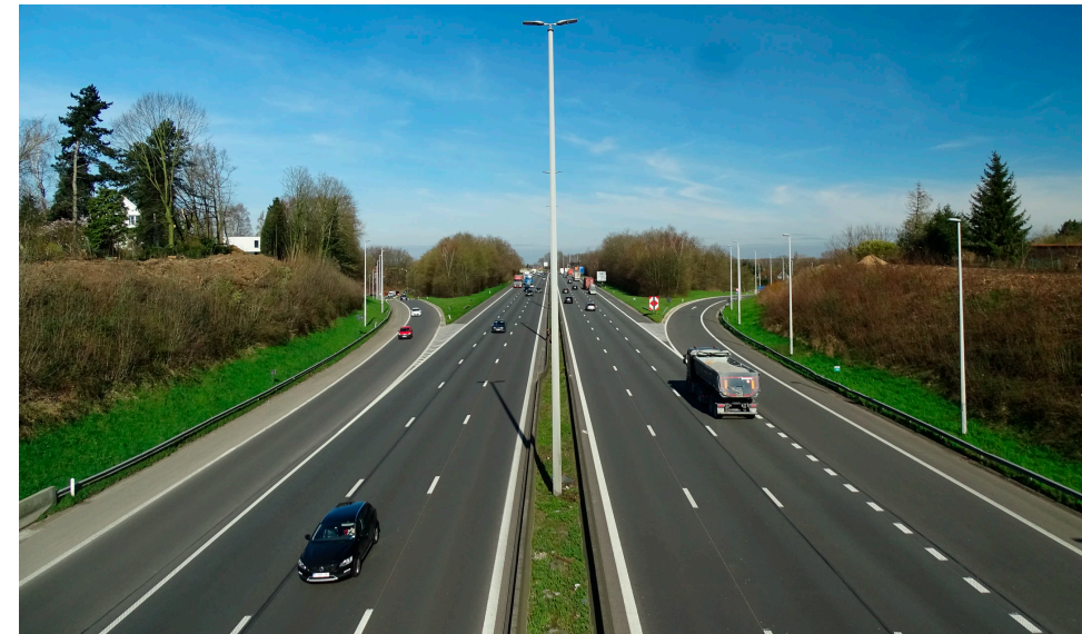
Highway HOV Lanes
